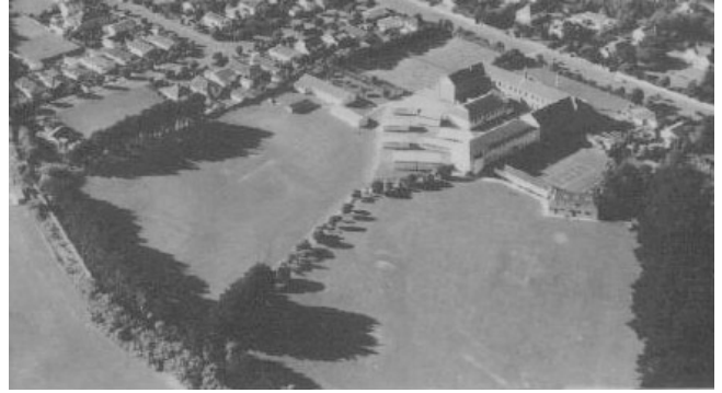
Aerial view of HVHS in 1956
